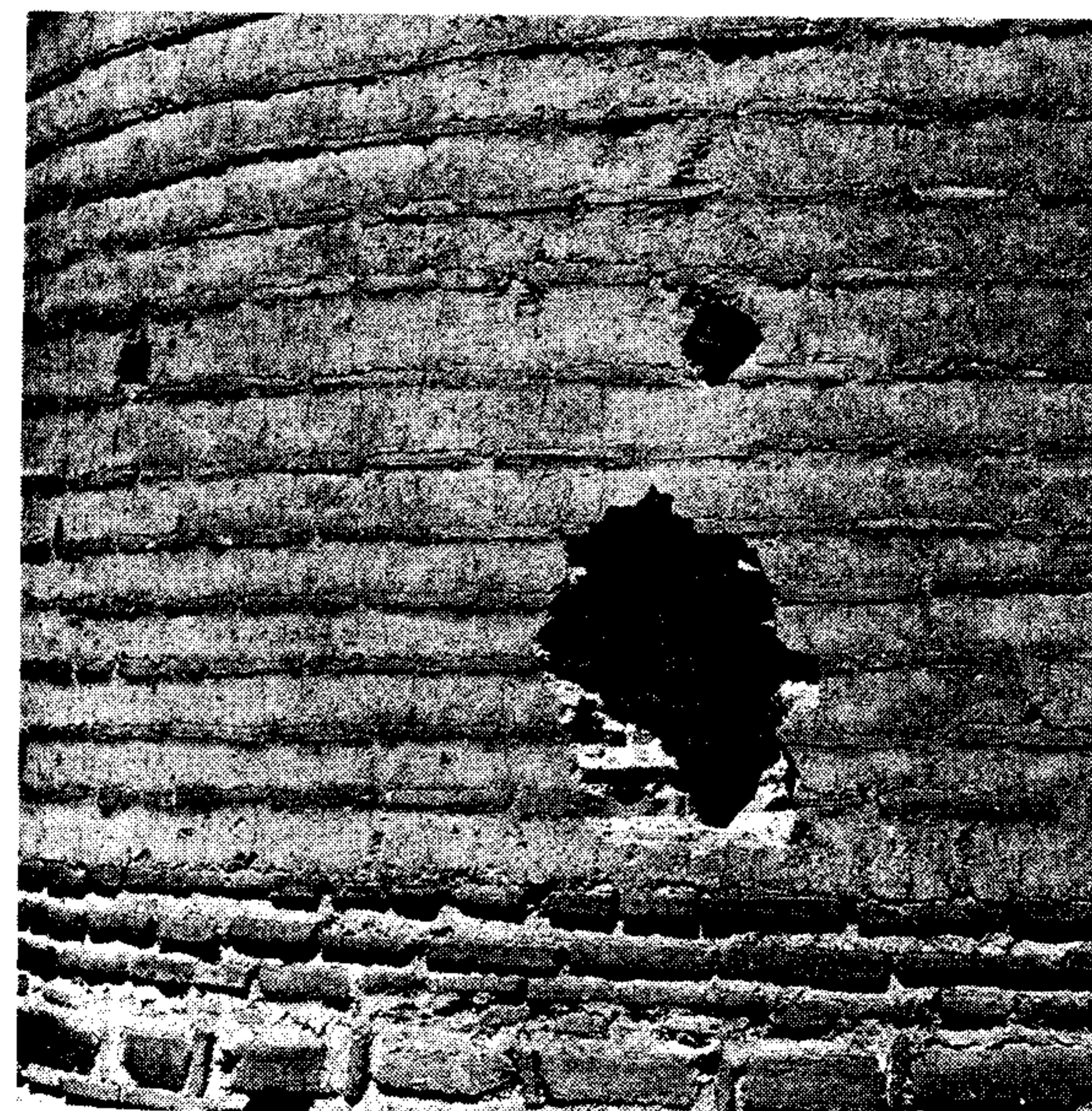
BRICKWORK TECHNIQUES AND PATTERNS. Recessed brick masonry; 11th C. Detail of the city walls of Nicaea.
